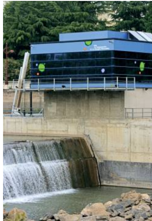
Micro hydropower installations have great chances of development.
