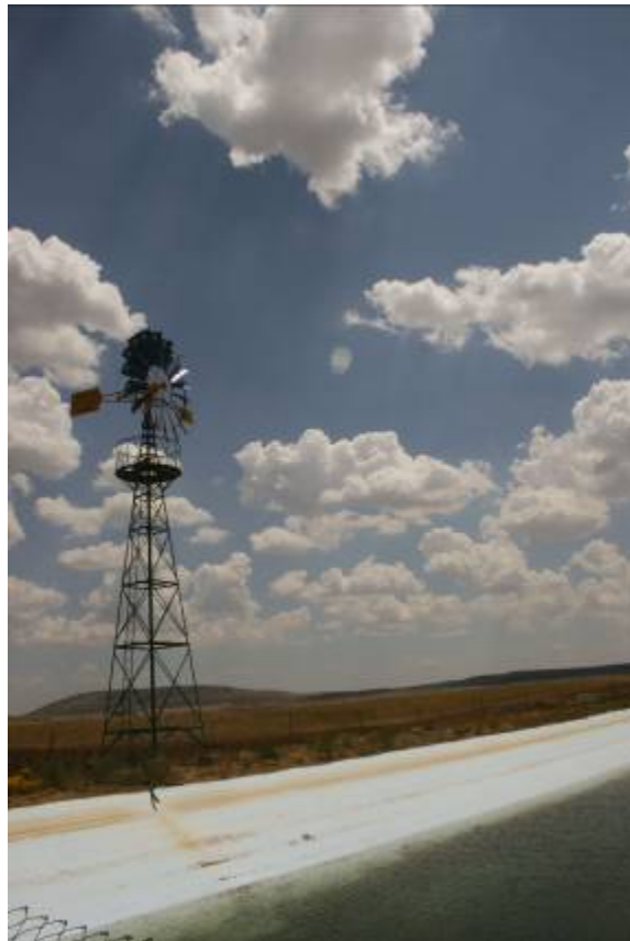
Wind power is an important alternative energy source.
